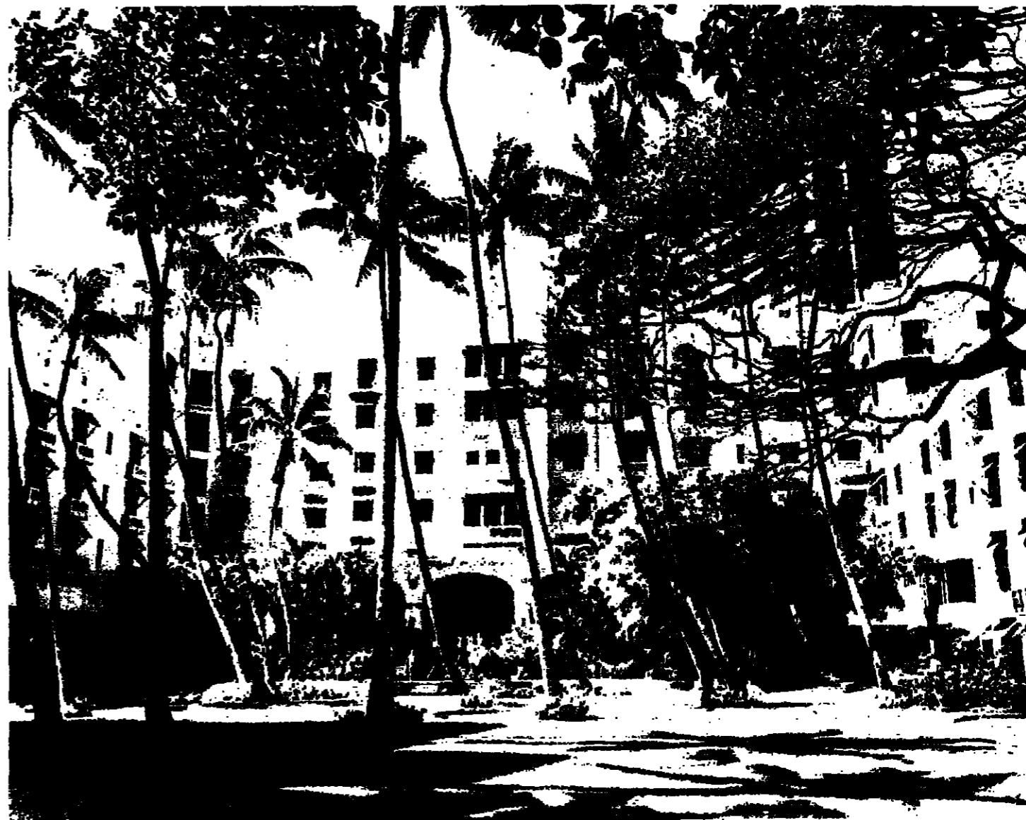
ROYAL HAWAIIAN: This hotel was originally created to be an elegant resort in the late 1920s. The 'Pink Palace' is curiously Moorish in style.
